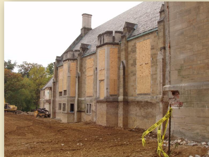
Rear View from North East
